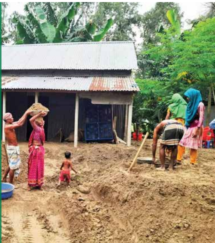
Lifting up the Homestead of a Beneficiary under ECCCP-Flood Project
